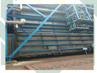
Gambar 2.3 Heat Recovery Steam Generator (HRSG)
