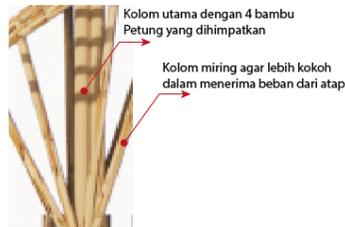
Gambar 4. 28 Detail Kolom
