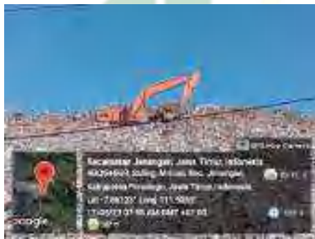
Gambar 4.5 Excavator TPA Mrican
