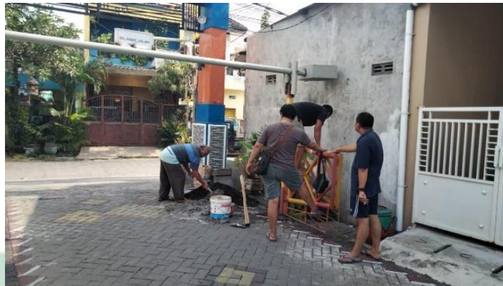
Gambar 4.4 Renovasi portal gang 3
