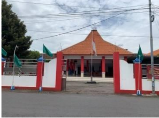
Gambar 5.5 Kantor Desa Balongdowo
